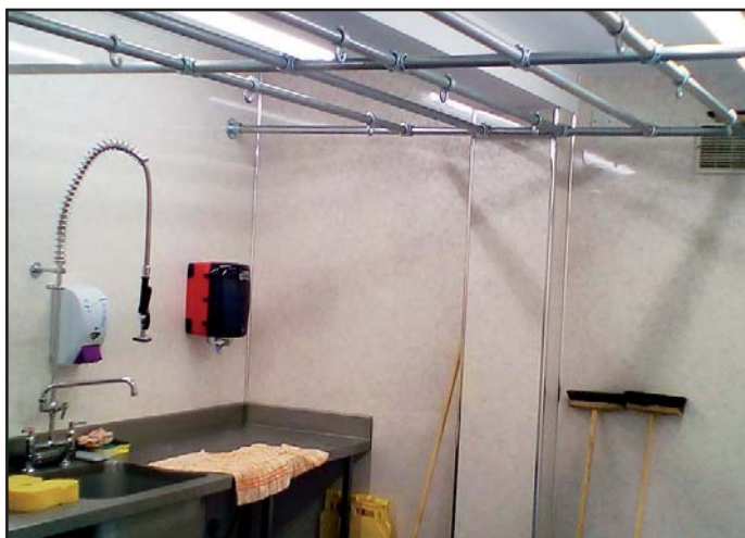
Plate 3: The integrated wet room with drying racks for kit washing and drying.
