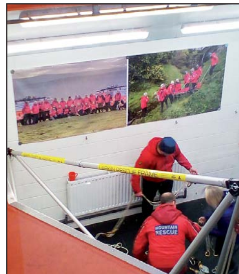
Right, Plate 4: The balcony with provision of belay anchorage to practice rope rigging and stretcher haulage.
